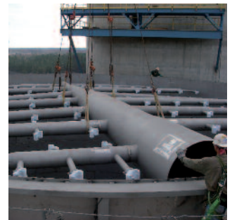
Customized configuration according state-of-art-technologies
