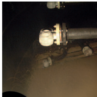
Customized configuration according state-of-art-technologies
